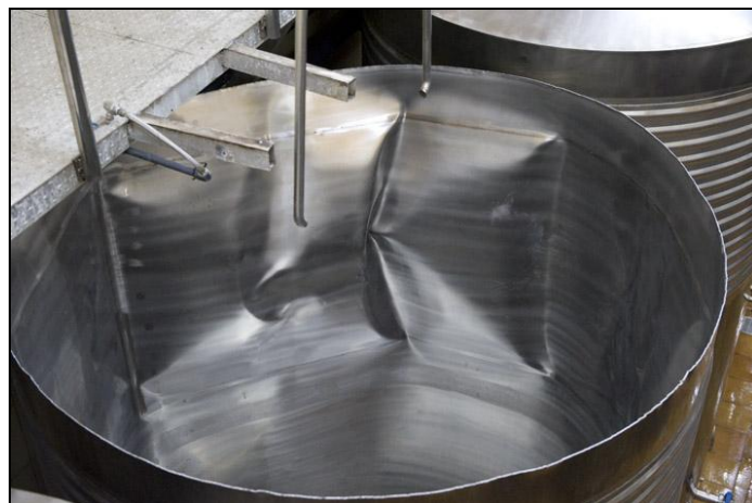
Once cut open for inspection the extent of the damage was clear to see
